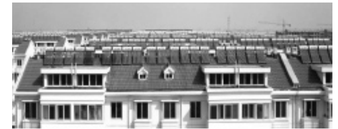
This European building is heated using renewable energy (notice panels on roof).
